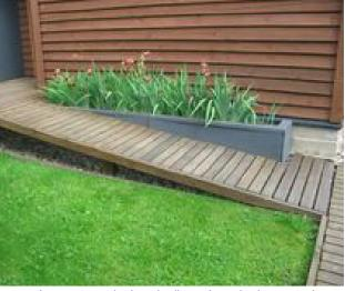
A 1:21 ramp does not require hand rails and can be integrated with landscaping
